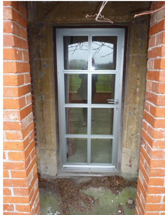
Figures 1 and 2 – Examples of the aluminium windows and doors installed prior to listing
