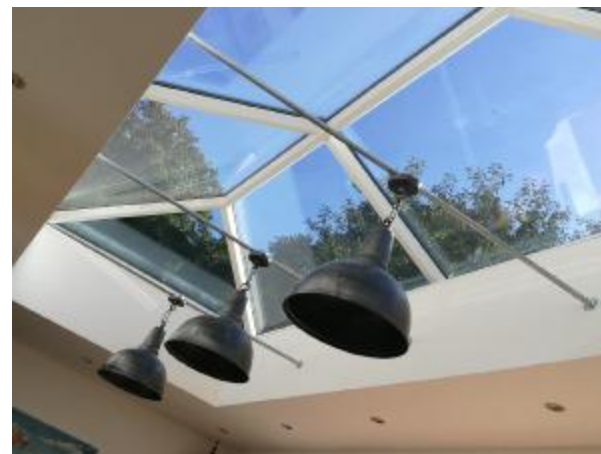
pyramid rooflight and lighting
