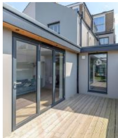
showing the box gutter and aluminium doors
